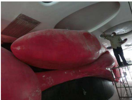
Figure 6. GRG module installation process.
